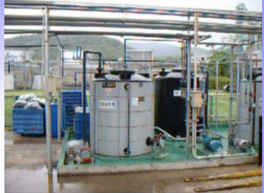
New Tank/Piping for Ethanol and Sugar Storage
